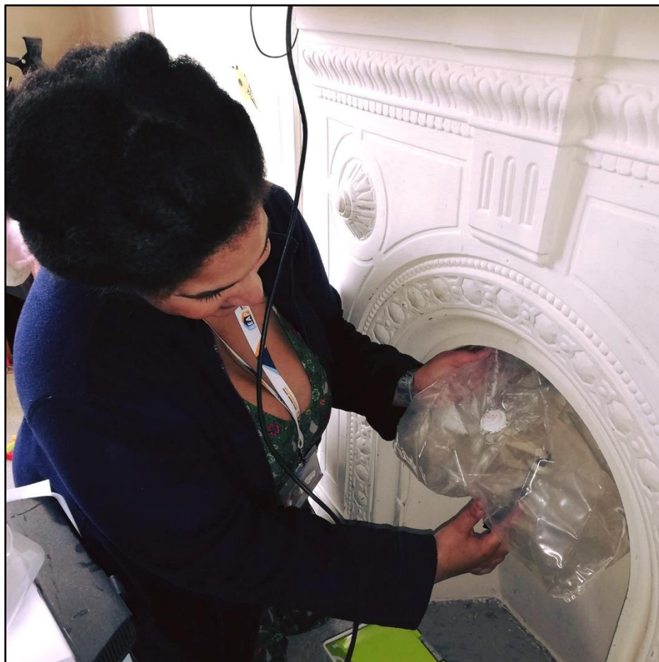
Picture: Fitting a heat saving 'chimney balloon'.
